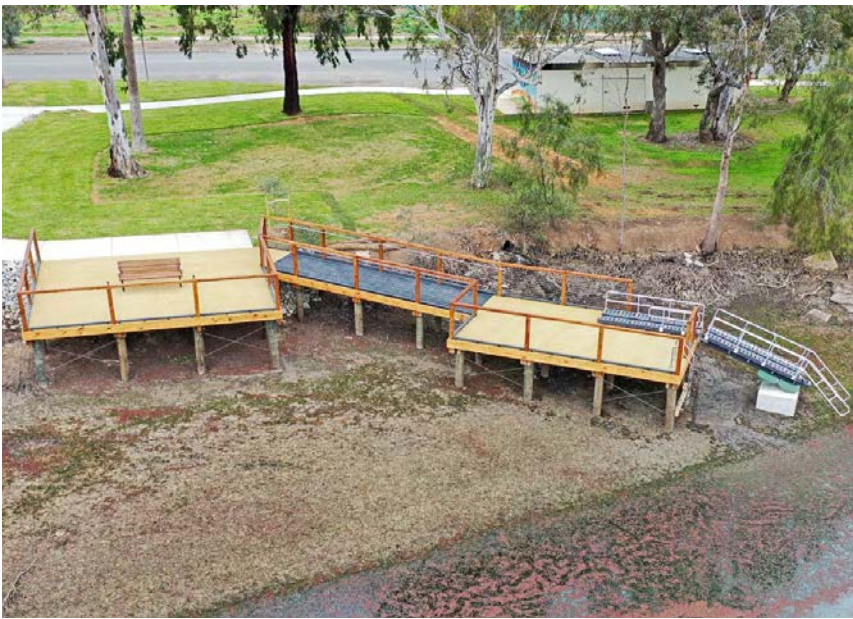
Lions Park, Gunbower - Fishing platform with ramp access to lower deck with accessible canoe launch (designed for fluctuating water levels)
