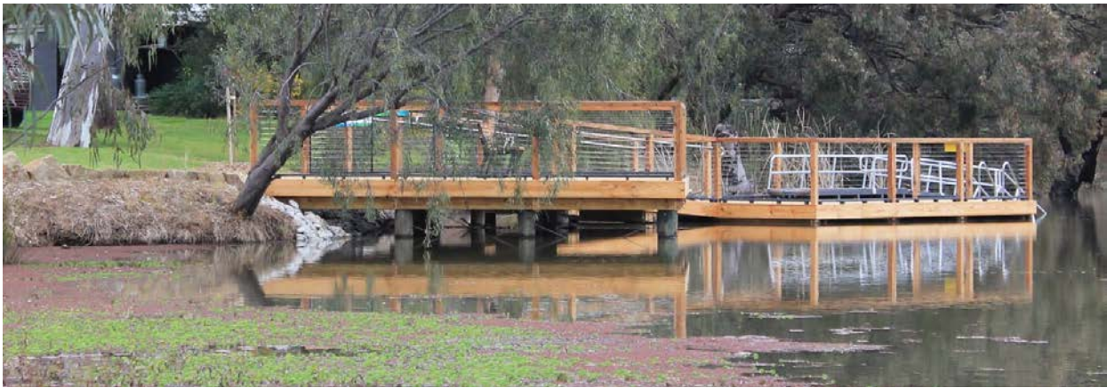
Lions Park, Gunbower - Fishing platform with ramp access to lower deck with accessible canoe launch (designed for fluctuating water levels)
