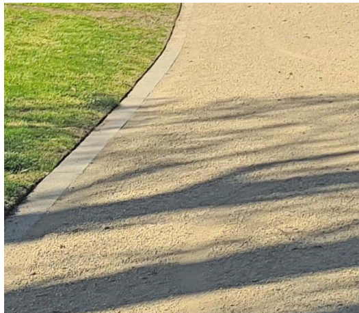
Compacted granitic sand & concrete edge shared path
