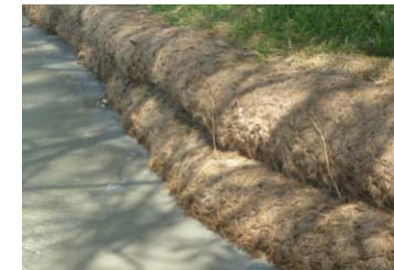
Coir log retaining wall
