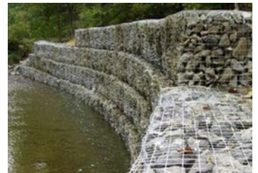
Gabion basket retaining wall
