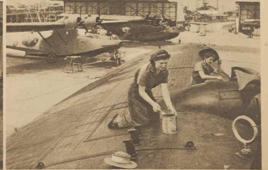
"DOPING" PATCHES on a flying-boat. Tarmac is right on the beach at this maintenance unit. Aircraft come direct from operational areas, often with bullet and shrapnel holes in fabric.
