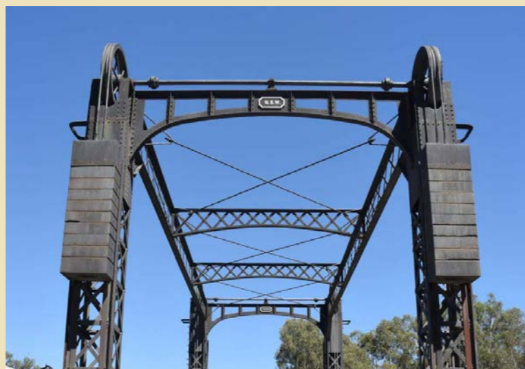
Cobram - Barooga Bridge, crisscross form in supports
