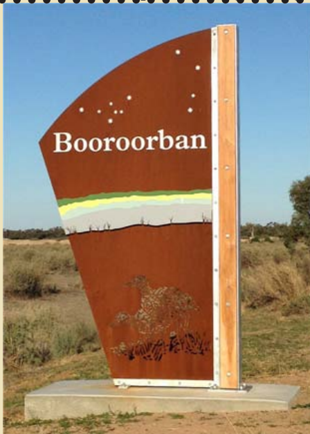
LMLA Booroorban entry sign with laser cut mild steel and layered two-pack paint panels
