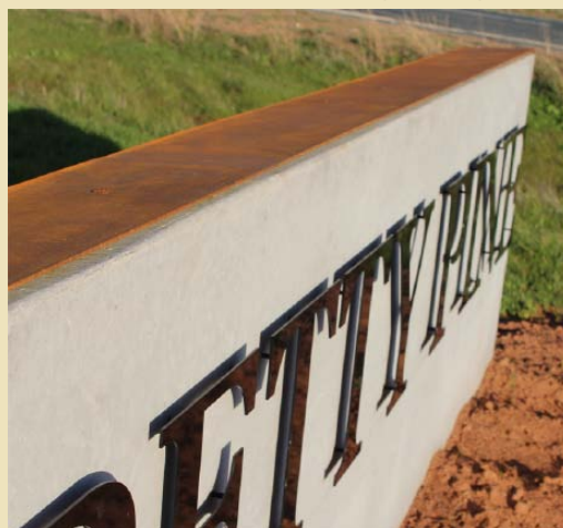
LMLA Pretty Pine entry sign with mild steel cap to concrete plinth
