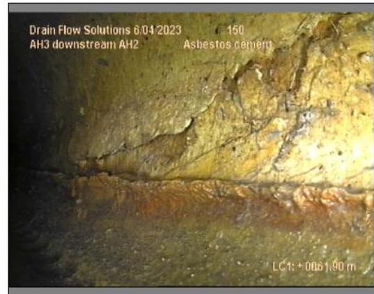
Photo: 5_1_7_06042023_130317_A.JPG 61.9m, Longitudinal fracture, width 100mm, General Comments Reline Required-Longitudinal cracking full length of pipe, at 3 o'clock
